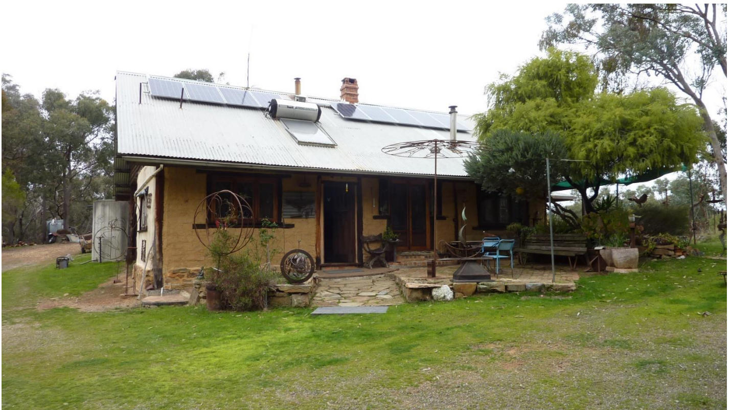
Photo 3 Looking south west towards the dwelling in the southern part of the site
