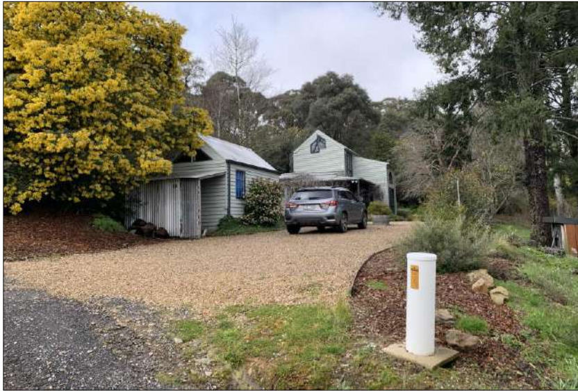
Existing dwelling on the site. Shed in the front that is to be demolished.
