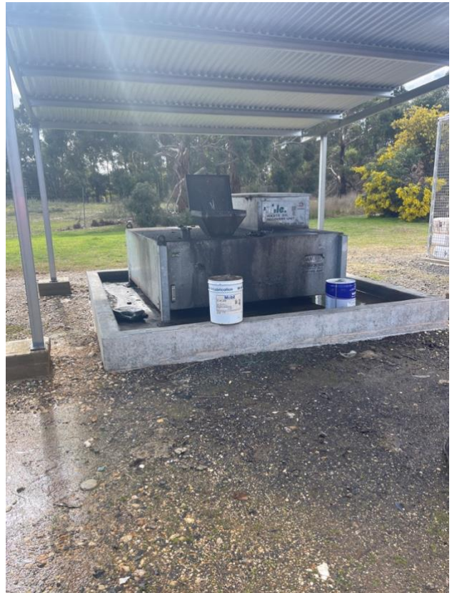
Waste oil area, drum of solvent store on bund edge
