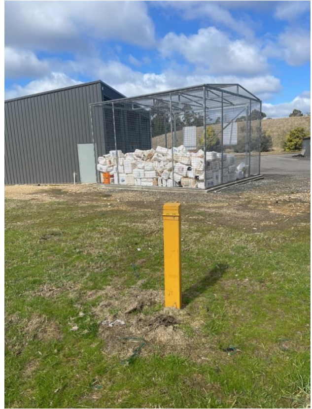
Drum muster cage and groundwater monitoring well
