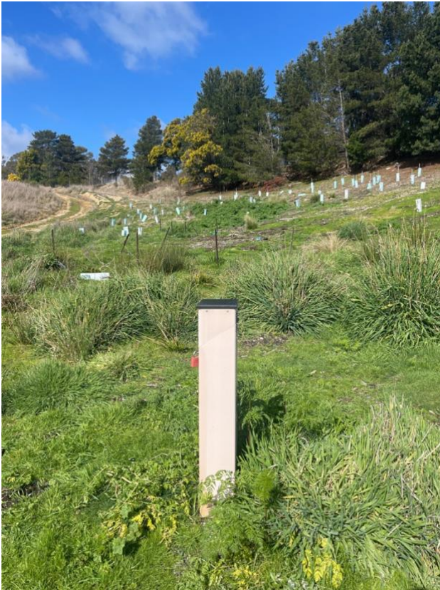
Groundwater monitoring well
