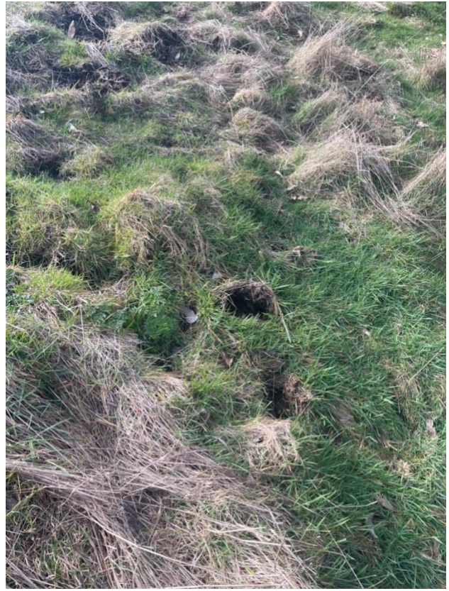
Evidence of animal burrowing within landfill cap
